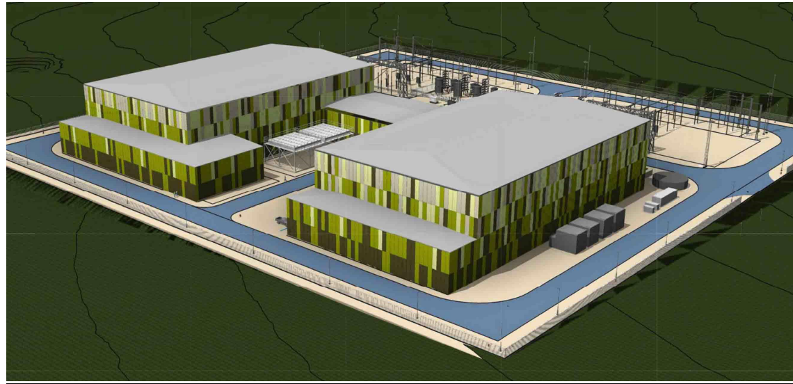
Plate 4.2- Green panels and hipped roofs
