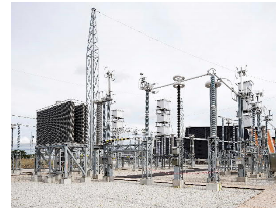
Plate 5.8 – Typical Lightning Masts Image: ©GE
