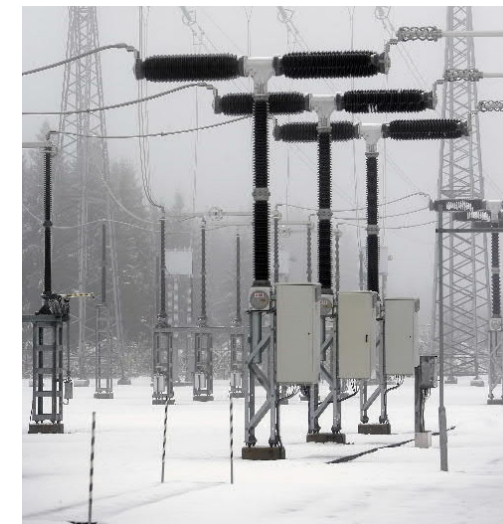
Plate 5.9 – Typical HVAC Circuit Breaker Image: ©ABB
