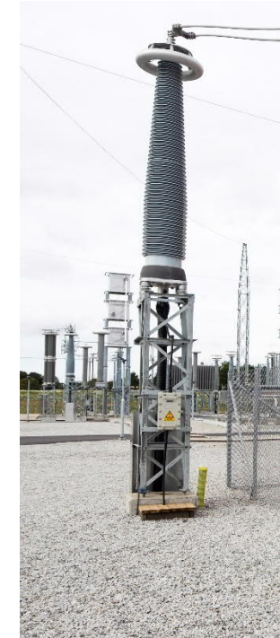
Plate 5.6 – Typical 400kV Cable Terminations Image: ©GE
