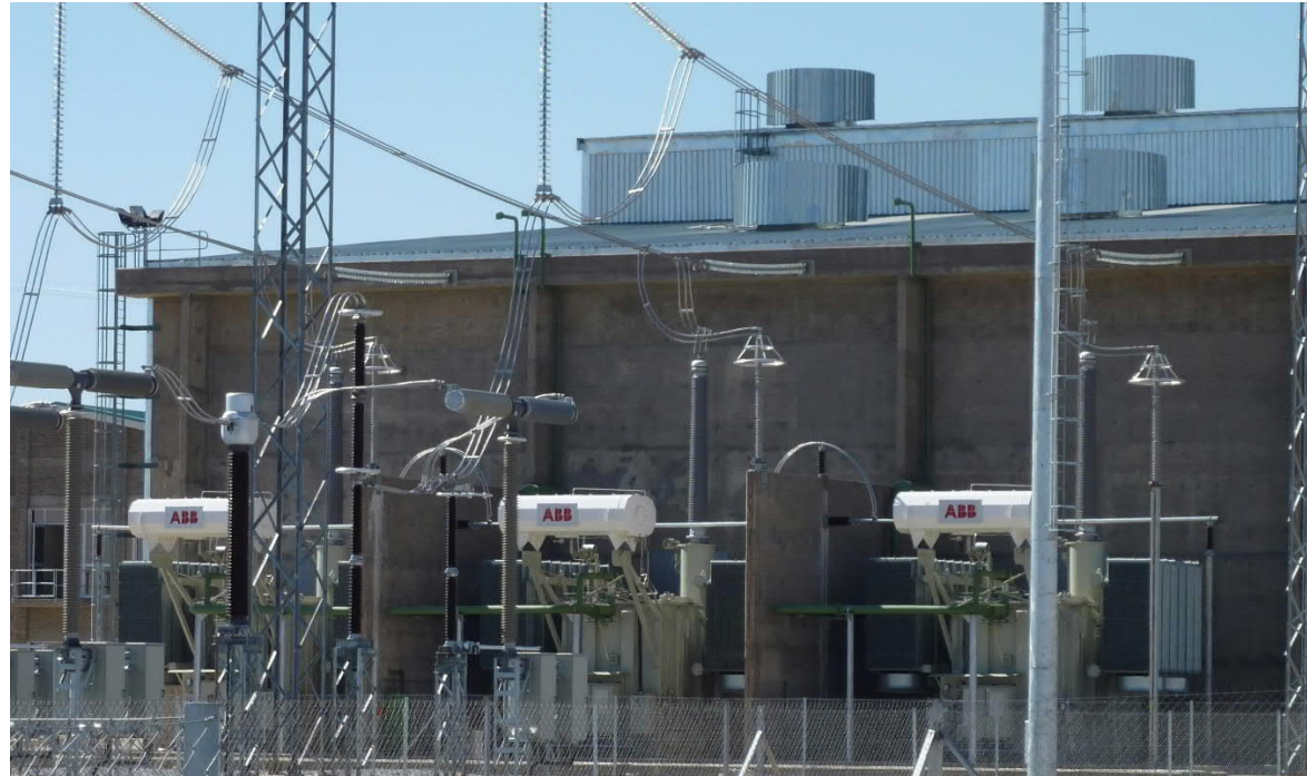
Plate 5.14 – Typical Interface transformers Image: ©ABB
