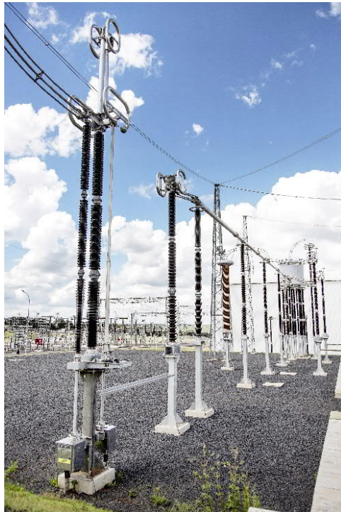
Plate 5.10 – Typical HVAC Disconnector Image: ©ABB
